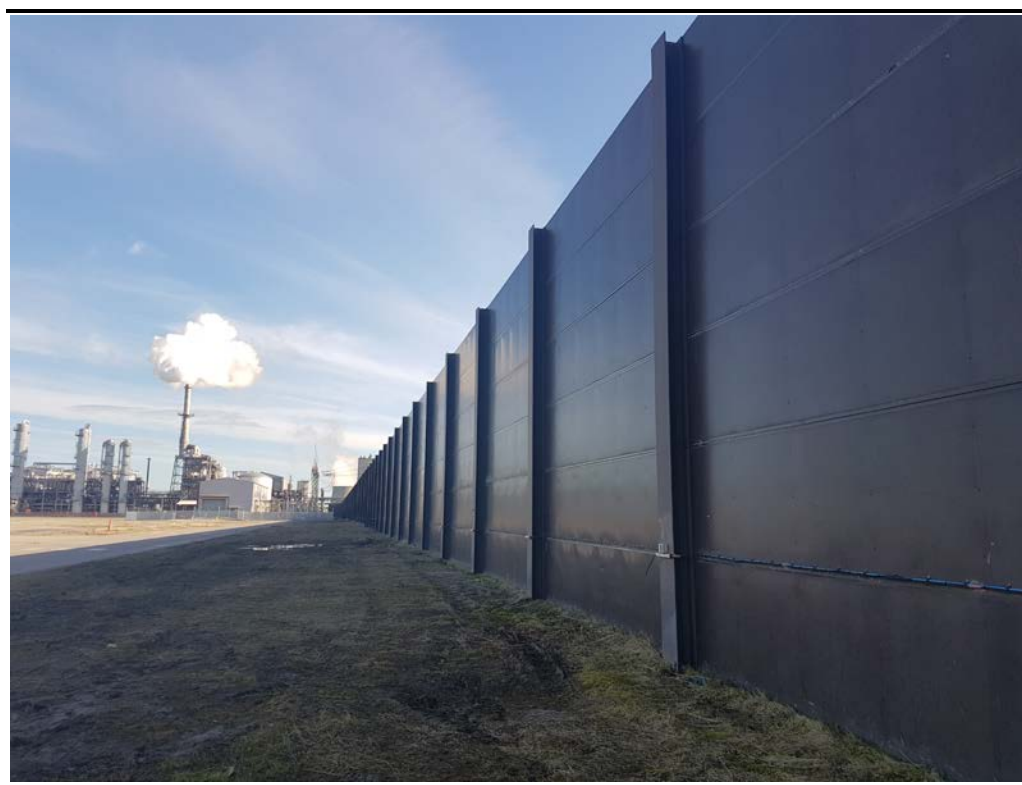
Figure 8.2 Existing Noise Wall to be Retained
